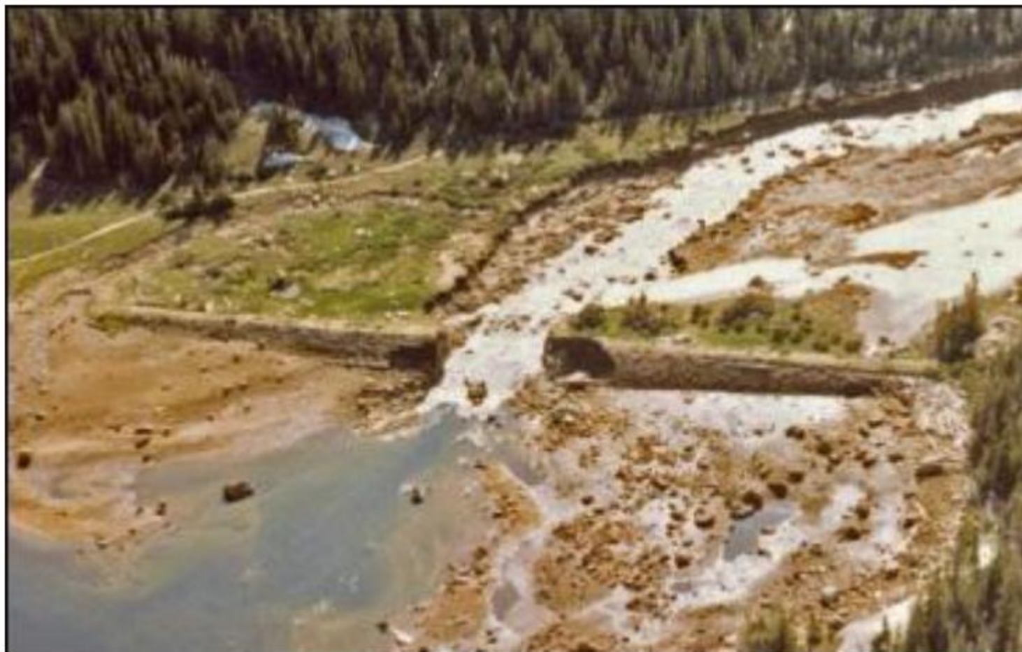
Figure 4: Aerial view of the dam breach [USBR photo]
