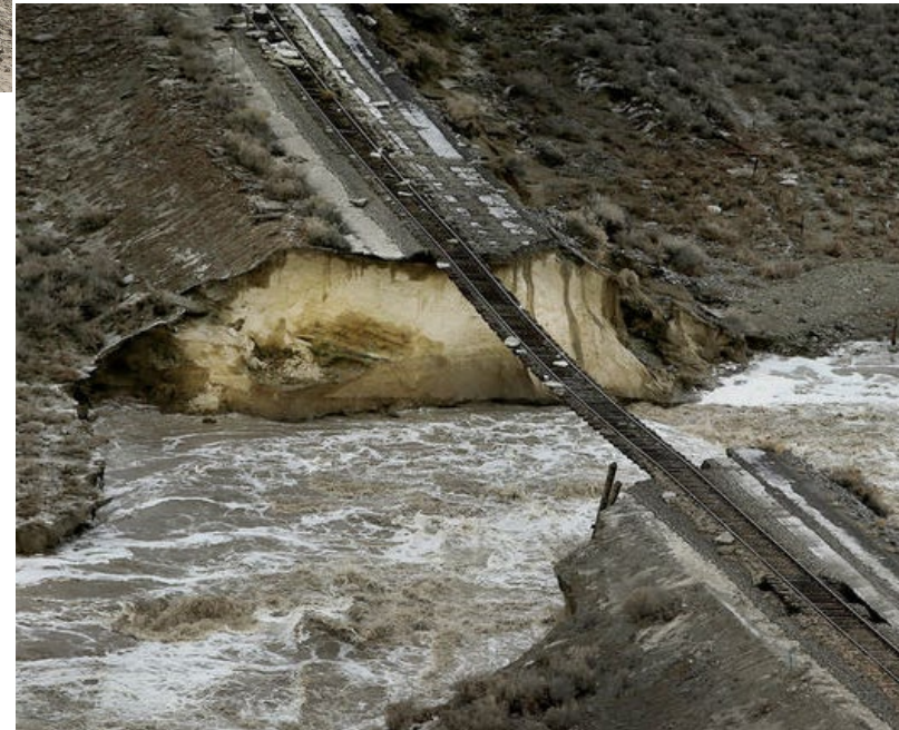
UPRR Railroad downstream of HWY 223
