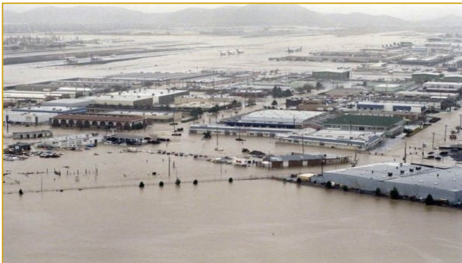
Sparks Industrial Park January 1, 1997, Flooding on the Truckee River.
